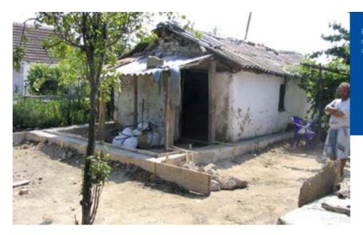
Photo 33: Foundations for a new house on the site of an old run-down one in Apatin
